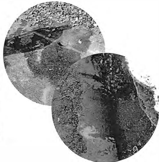
Leak on AC Main Line
