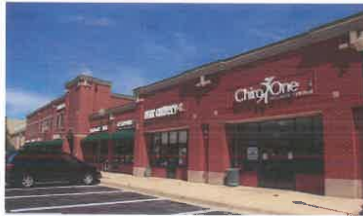
Figure C9.1a: Scale of signage is appropriate for building. Multiple signs are displayed in a consistent manner.
