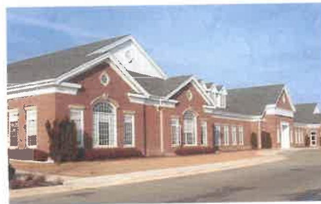
Figure A2.2b: This building uses varied roof forms and façade planes to reduce apparent size.
