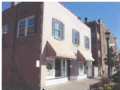
Fig. 40: It is important to provide details at the top of buildings. In this example, the parapet does not have any detail or cornice. Buildings without detail at the top should be avoided
