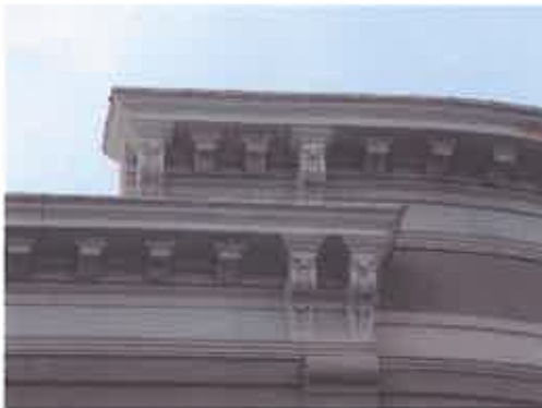
Fig. 37: Encouraged: cornice detailing
