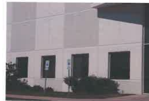
Figure C5.3.iva: Surface texture and detailing used to reduce building massing
