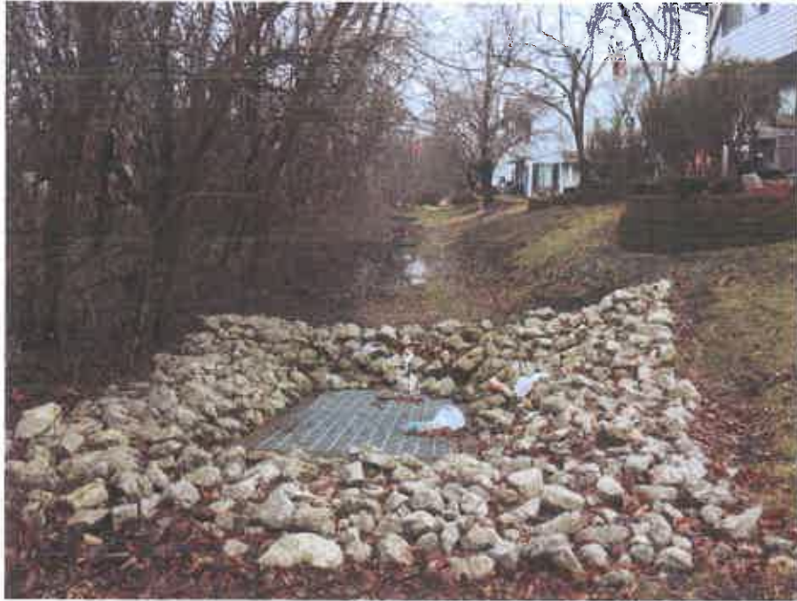
Storm Sewer Discharge into Sawmill Creek Reach No. 8
