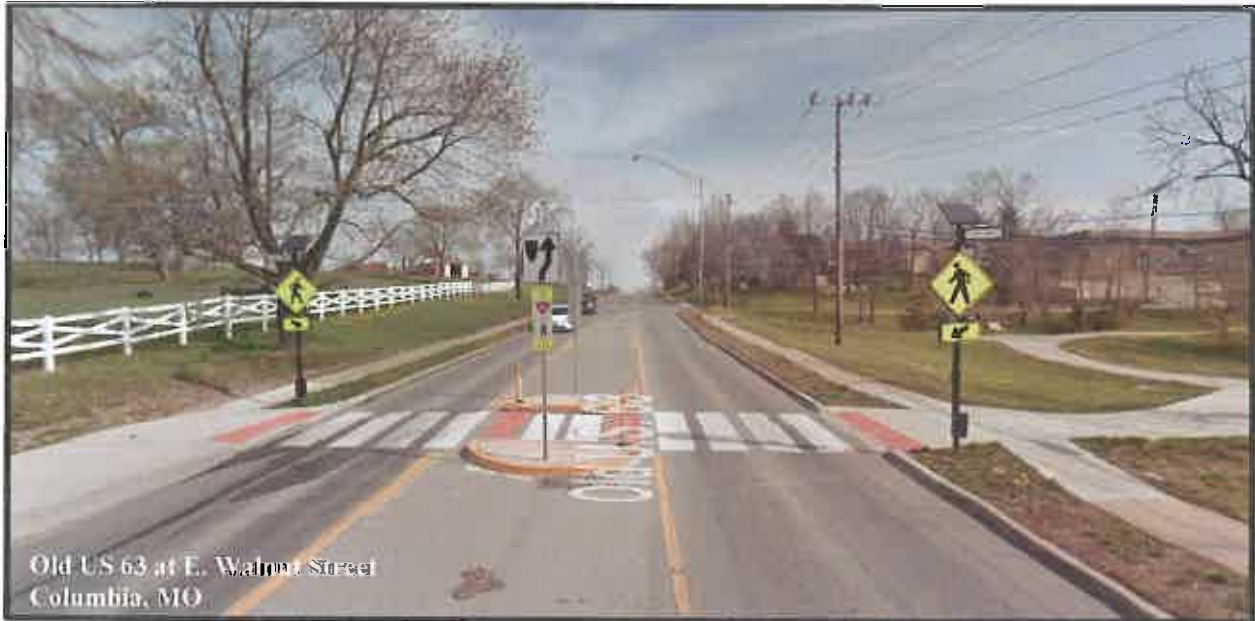
Figure 12 Example of Recommended Midblock Pedestrian Crossing Treatment
