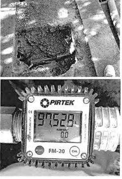
Pipe Info: 100mm (4 in.) PVC main & 20mm (0.75 in.) poly road conduit Correlation Score: 100% Logger Spacing: 77.4m (254 ft)
