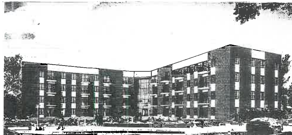
VIEW FROM SOKOL COURT
