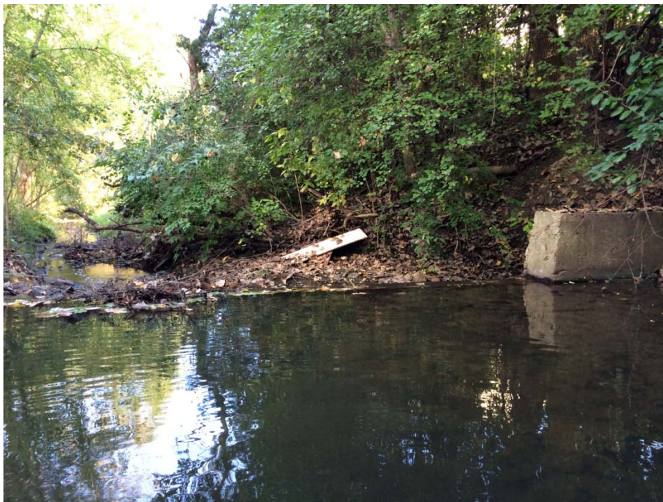
Photo No. 8 – Weir Downstream
