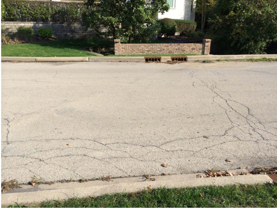
Photo No. 3 – Roadway (looking east)
