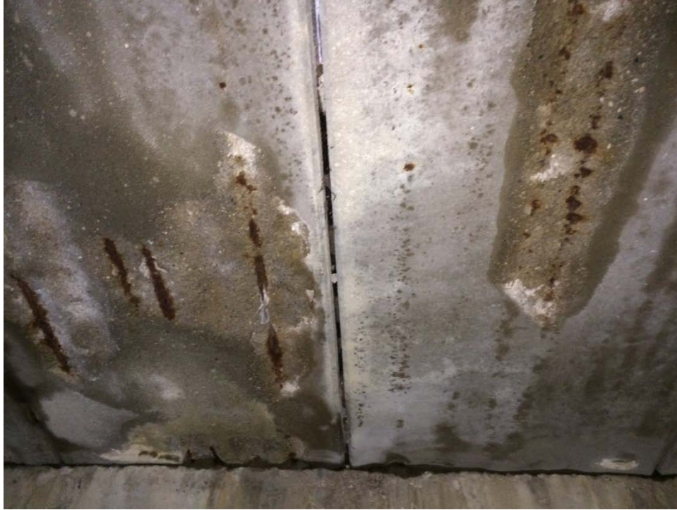
Photo No. 5 – Underside Precast Panels
