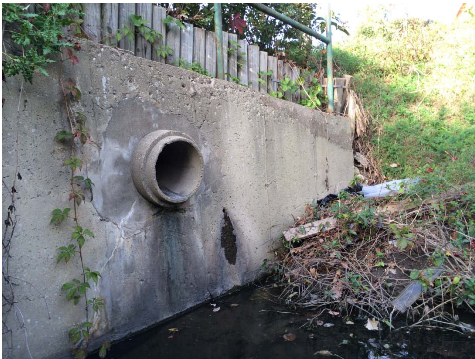
Photo No. 8 – Pipe Penetration
