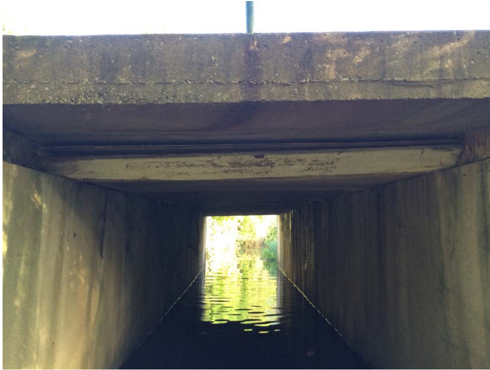
Photo No. 1 – Inside of Culvert
