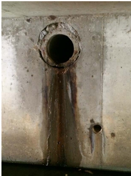
Photo No. 6 – Pipe Penetration
