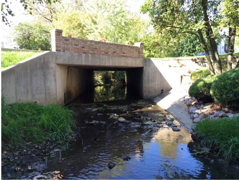
Photo No. 1 – East Elevation
