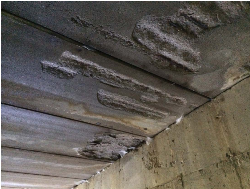
Photo No. 6 – Underside Precast Panels
