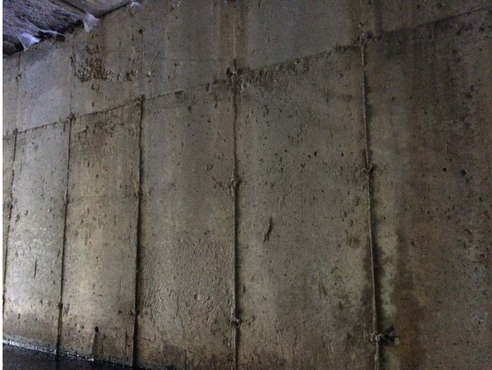
Photo No. 7 – Typical Wall Condition
