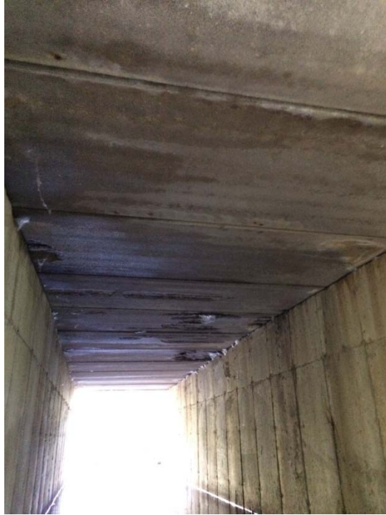
Photo No. 1 – Inside of Culvert
