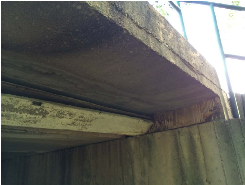
Photo No. 6 – Cast-in-place “sidewalk” on each end
