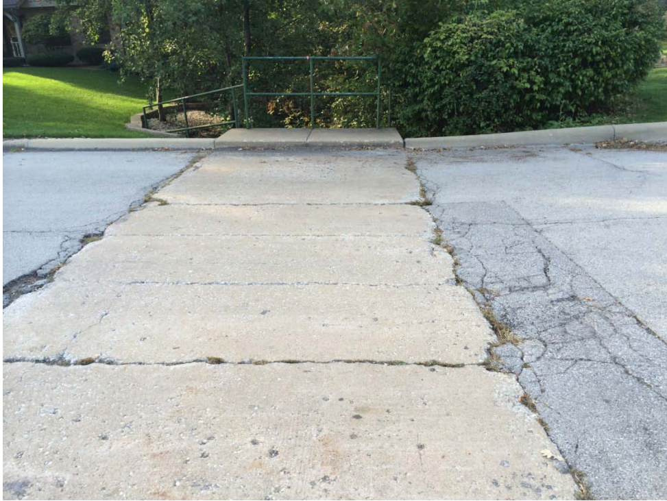
Photo No. 3 – Roadway Surface
