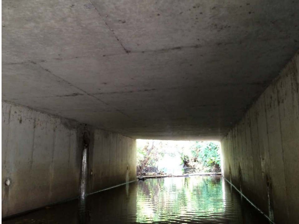
Photo No. 7 – Inside of Culvert
