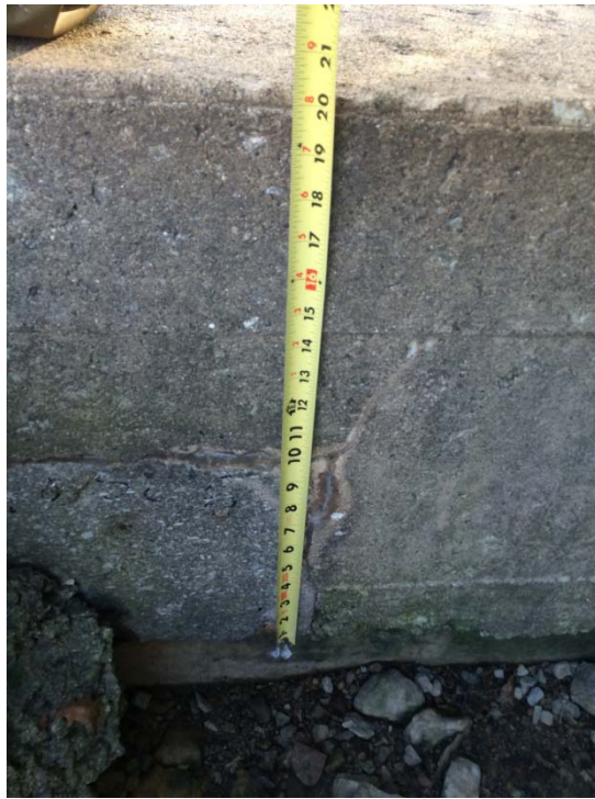
Photo No. 4 – Concrete Thicknesses
