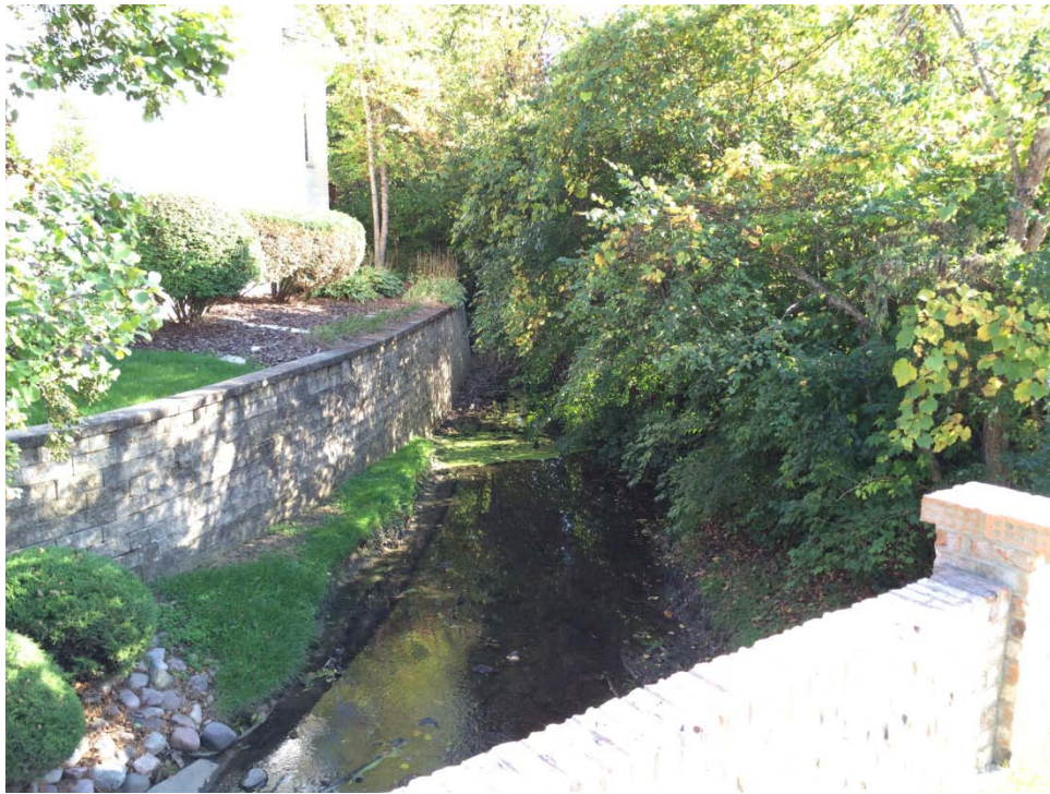
Photo No. 4 – Looking Downstream (looking east)
