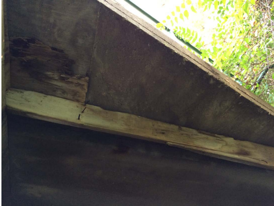
Photo No. 7 – Cast-in-place “sidewalk” on each end
