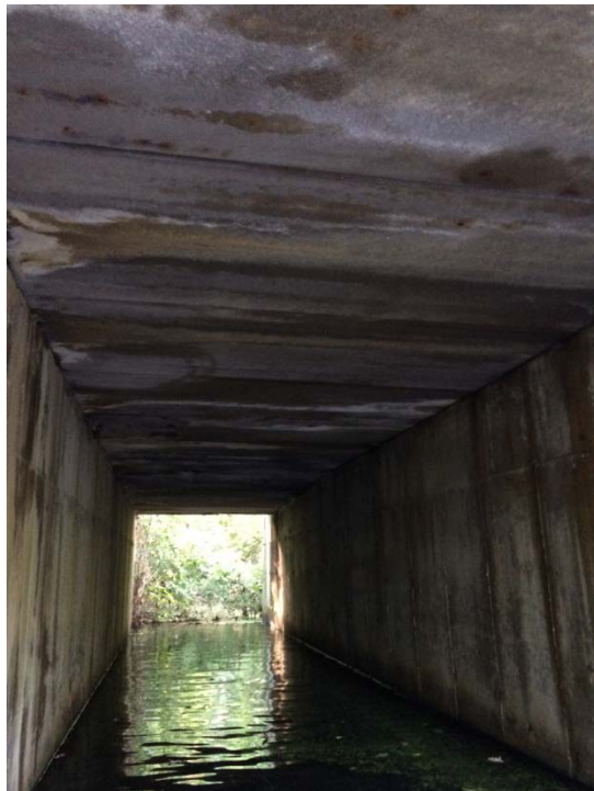
Photo No. 2 – Inside of Culvert
