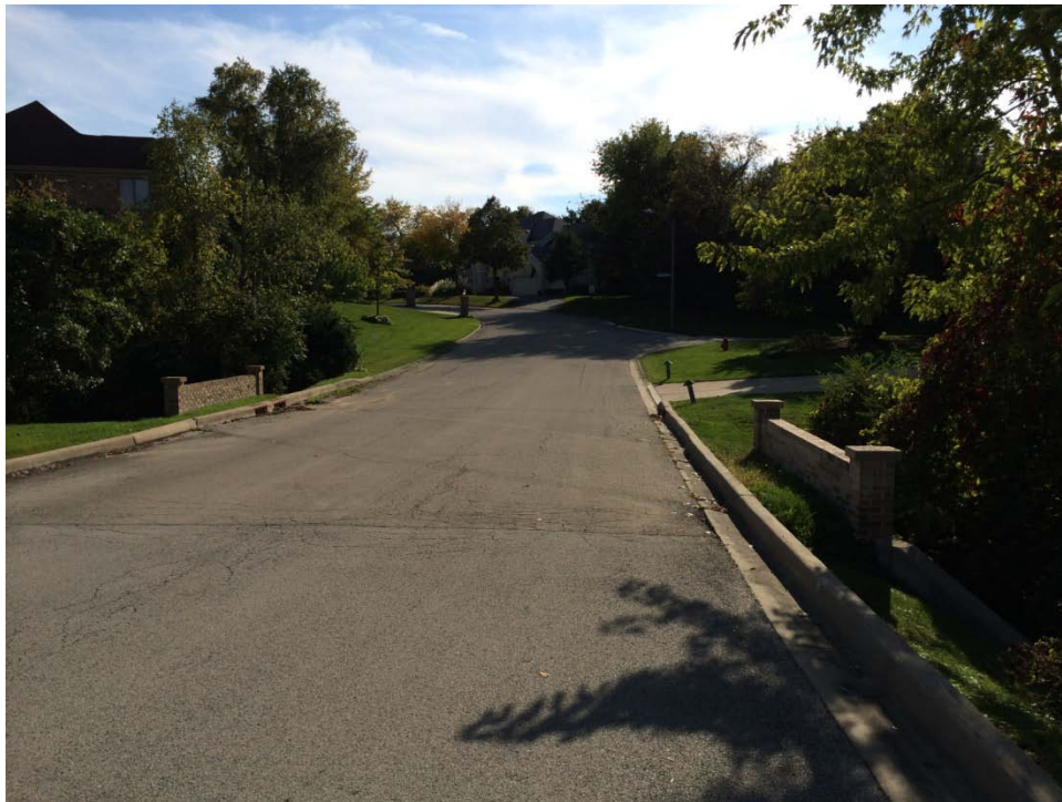
Photo No. 2 – Roadway Above (looking south)
