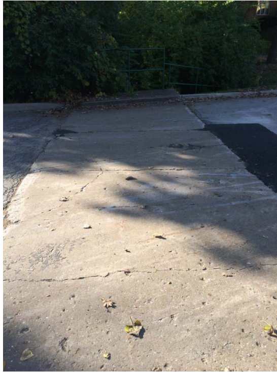
Photo No. 3 – Roadway Surface
