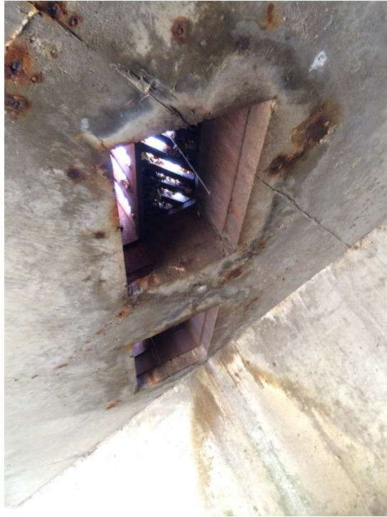
Photo No. 5 – Drains
