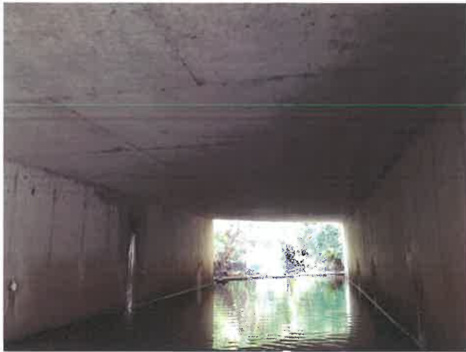
Photo No. 7 -- Inside of Culvert
