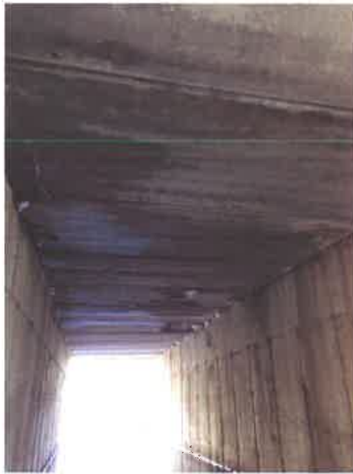
Photo No. 1 – Inside of Culvert
