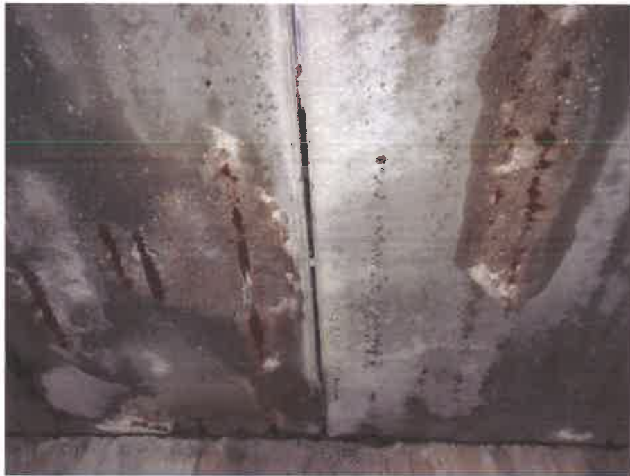
Photo No. 5 – Underside Precast Panels
