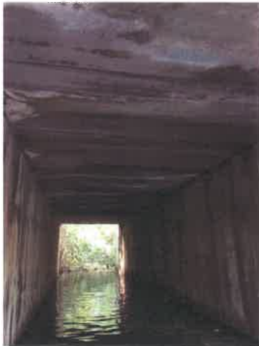
Photo No. 2 – Inside of Culvert
