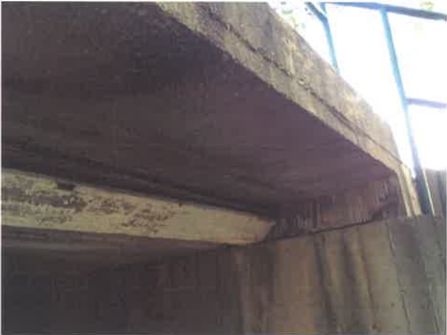
Photo No. 6 – Cast-in-place "sidewalk" on each end
