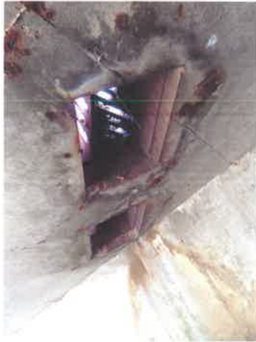
Photo No. 5 – Drains
