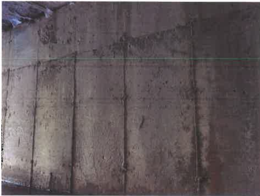
Photo No. 7 – Typical Wall Condition
