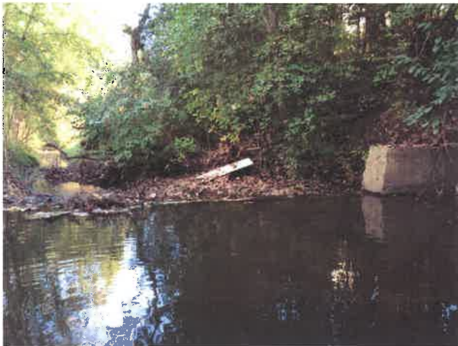
Photo No. 8 – Weir Downstream
