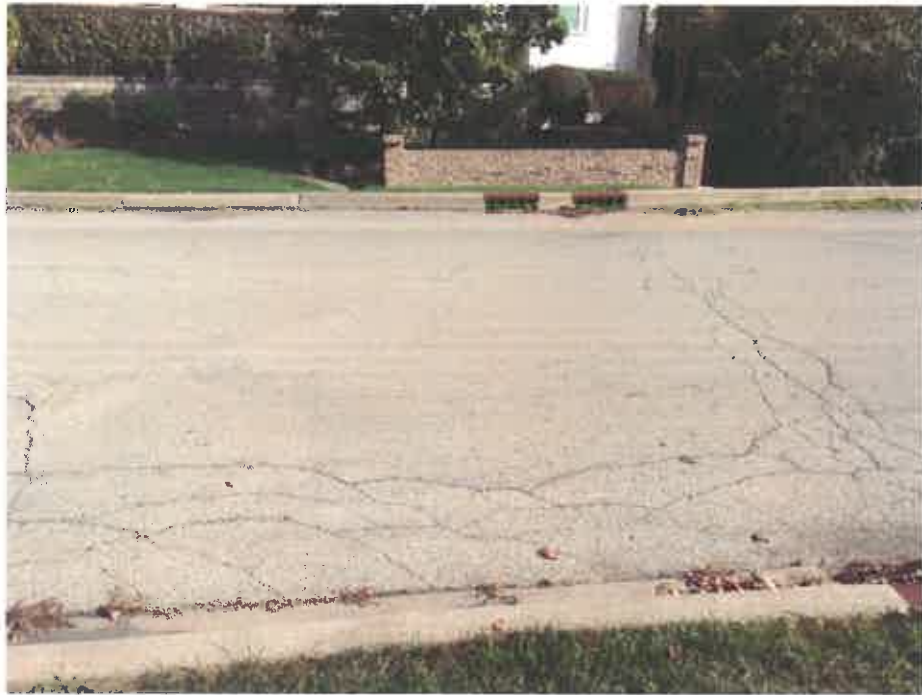
Photo No. 3 – Roadway (looking east)
