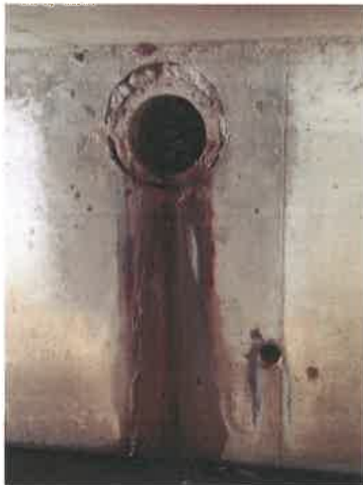
Photo No. 6 – Pipe Penetration
