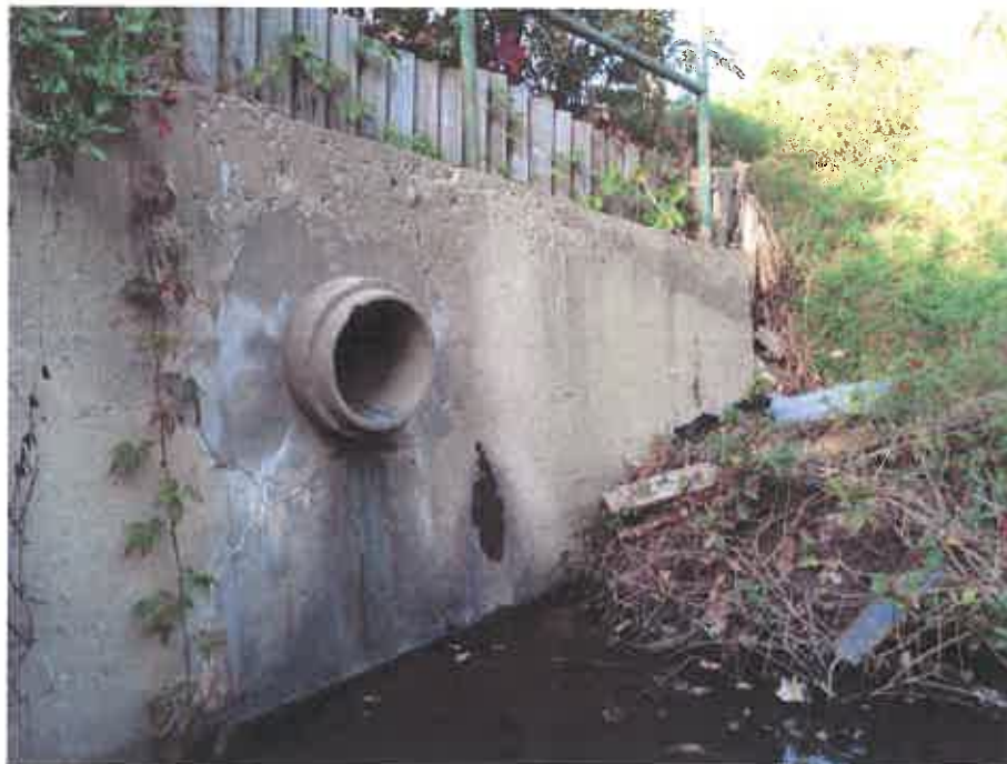
Photo No. 8 – Pipe Penetration
