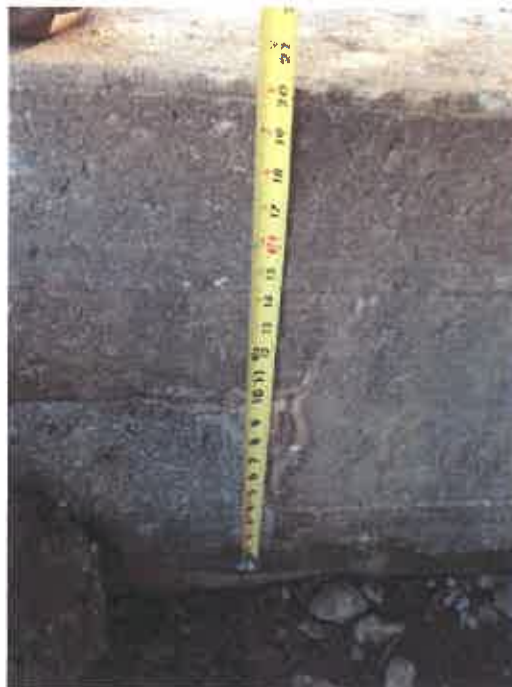
Photo No. 4 – Concrete Thicknesses
