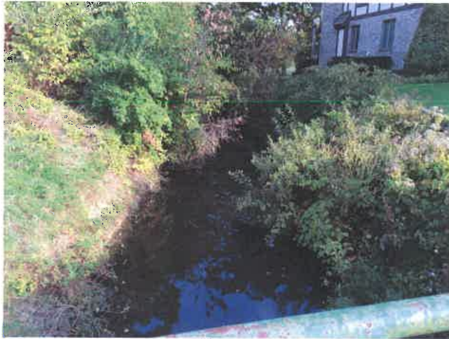
Photo No. 7 – Looking Downstream
