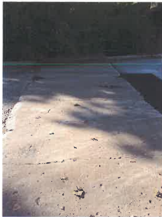
Photo No. 3 – Roadway Surface
