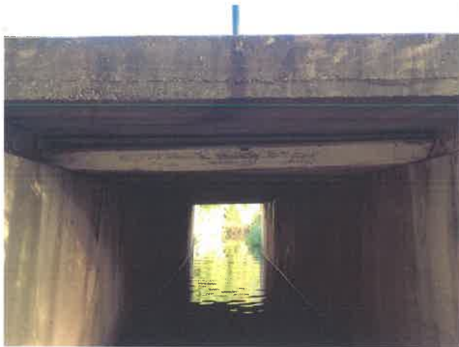
Photo No. 1 – Inside of Culvert
