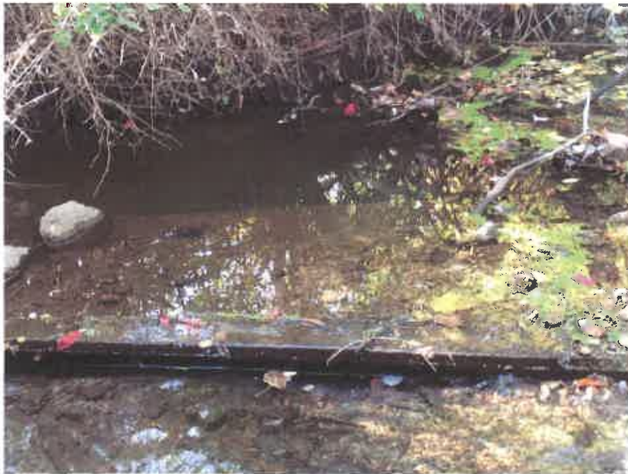
Photo No. 8 -- Weir Upstream End
