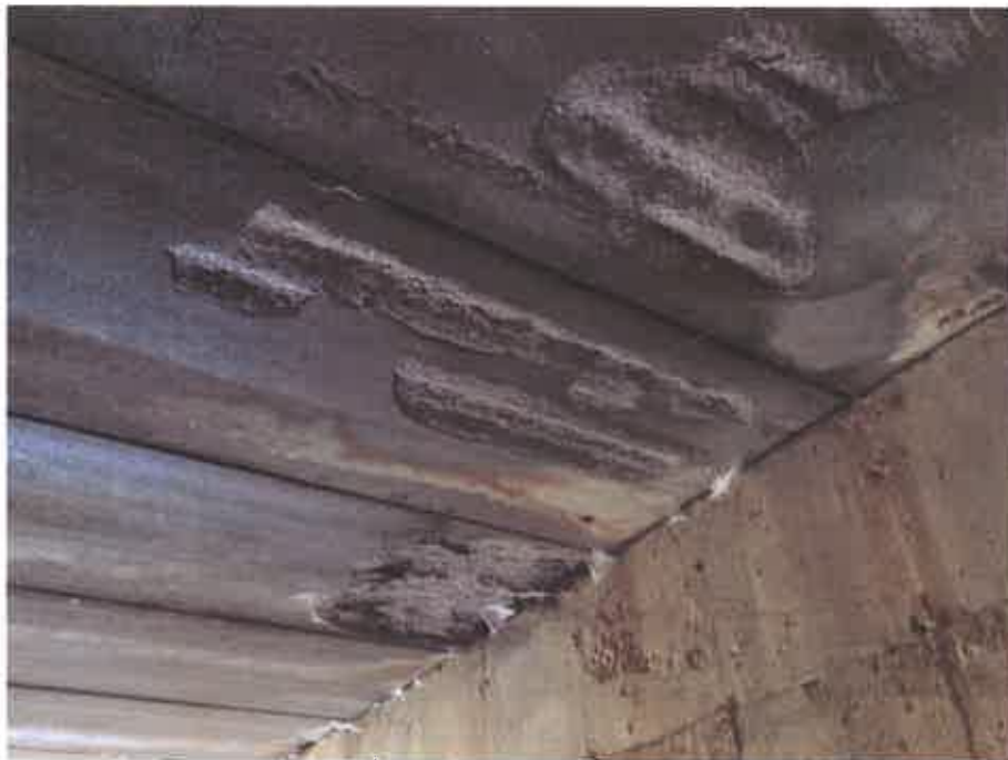
Photo No. 6 – Underside Precast Panels
