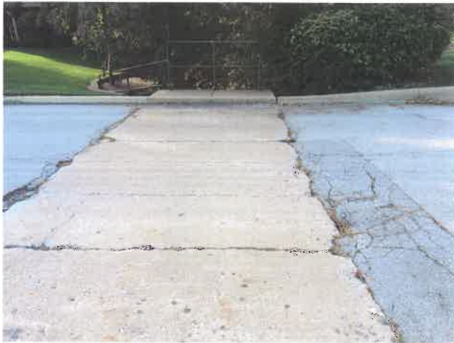
Photo No. 3 – Roadway Surface
