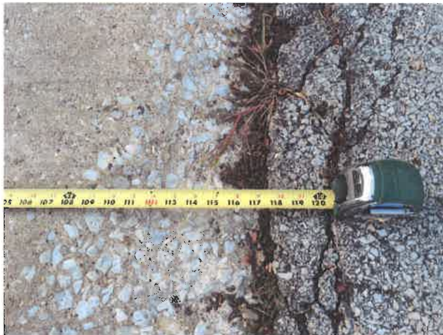
Photo No. 8 – Concrete Width
