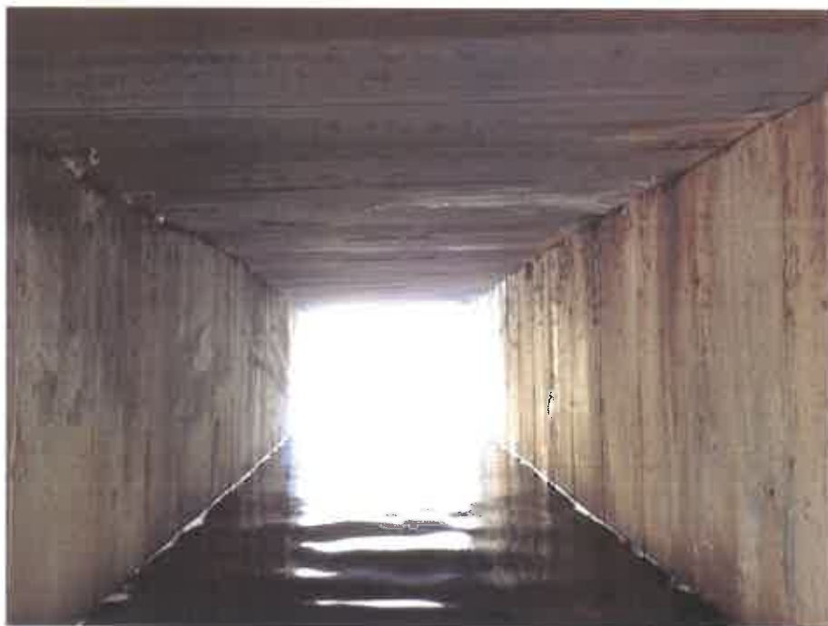
Photo No. 2 – Inside of Culvert
