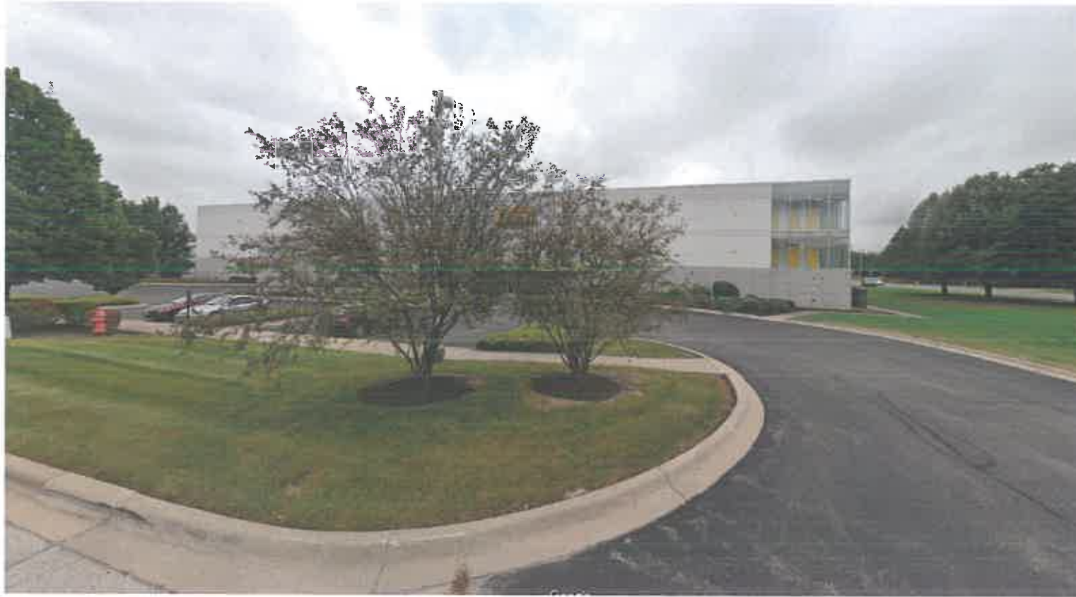
View from North Side of Building
