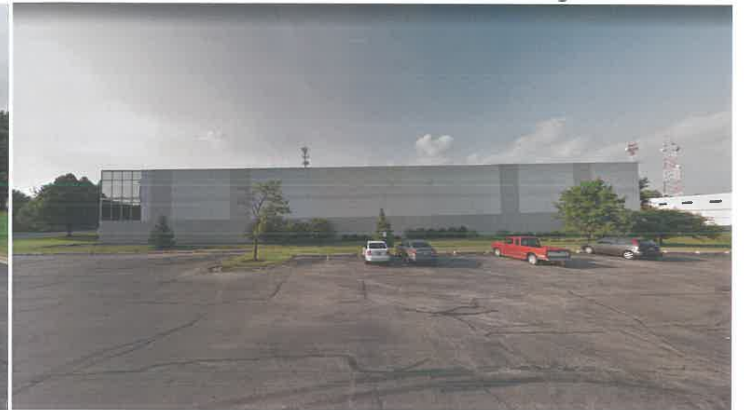
View from South Side of Building
