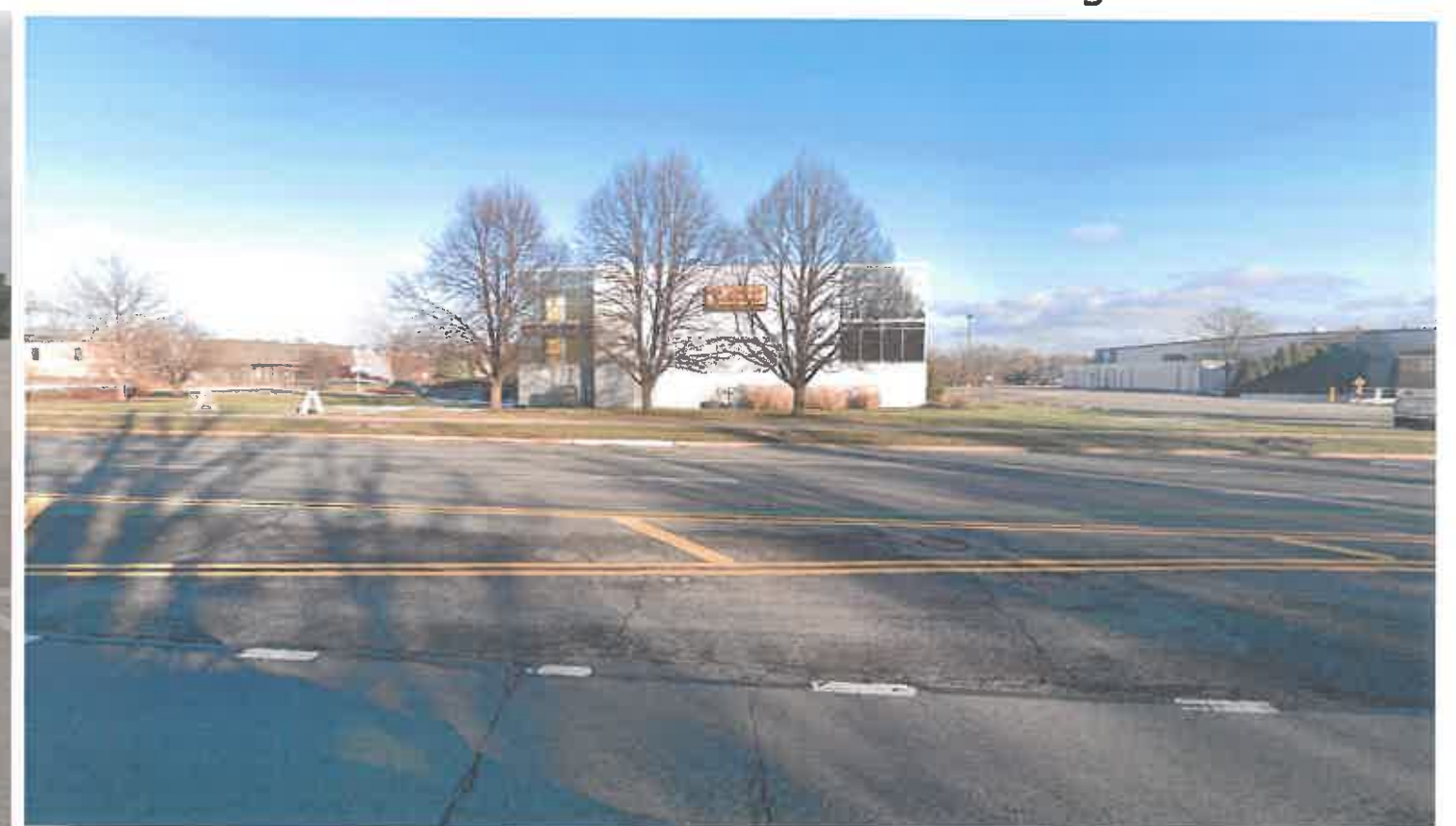
View from West Side of Building
