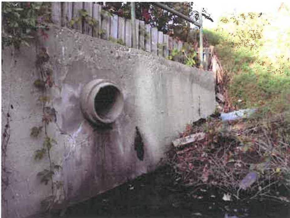
Photo No. 8 – Pipe Penetration
