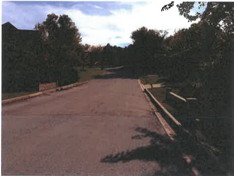
Photo No. 2 – Roadway Above (looking south)
