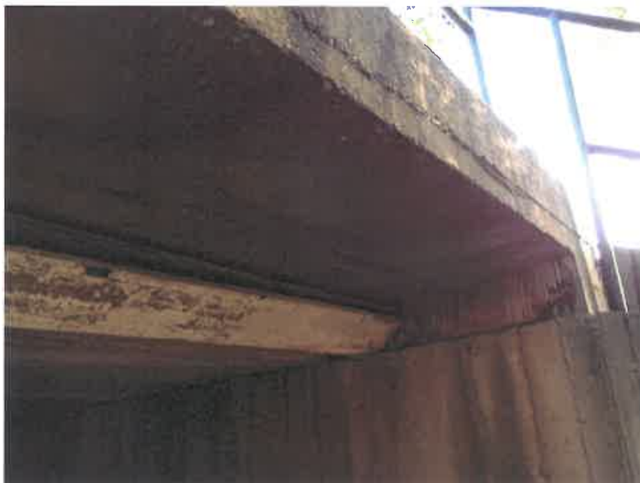
Photo No. 6 – Cast-in-place "sidewalk" on each end
