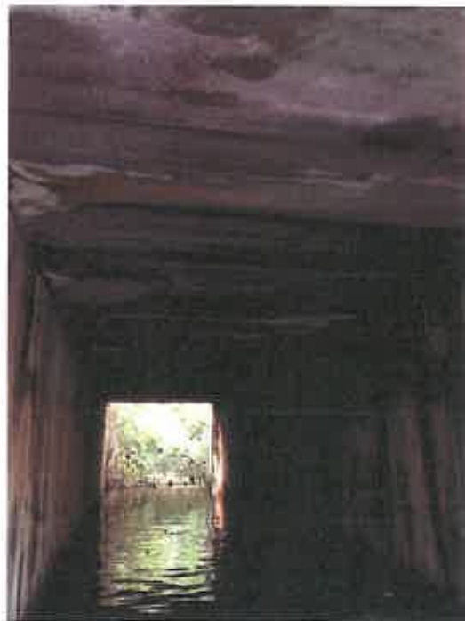
Photo No. 2 – Inside of Culvert
