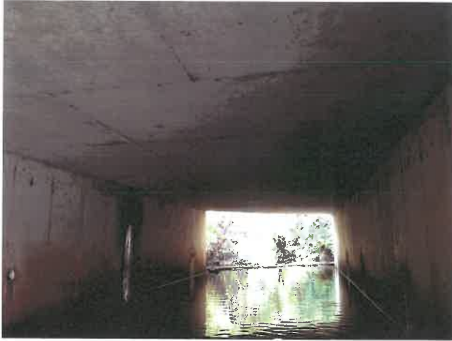
Photo No. 7 – Inside of Culvert
