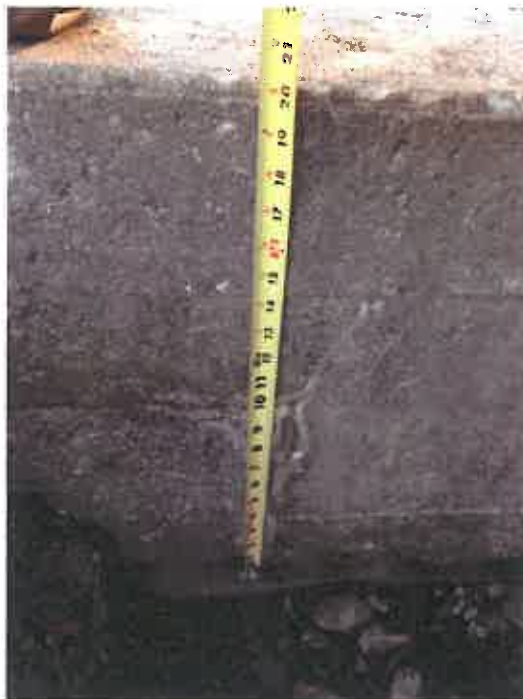
Photo No. 4 – Concrete Thicknesses
