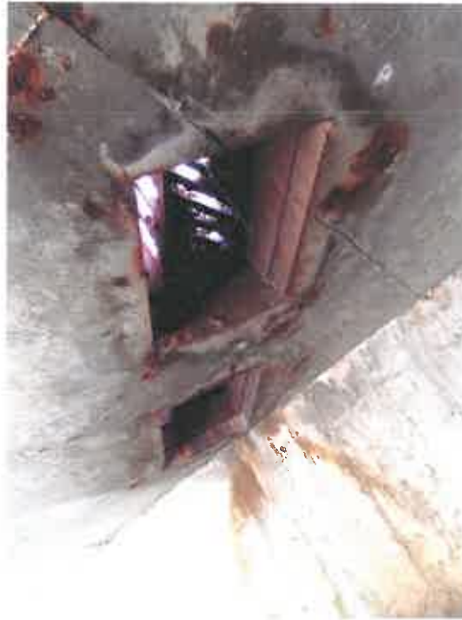
Photo No. 5 – Drains
