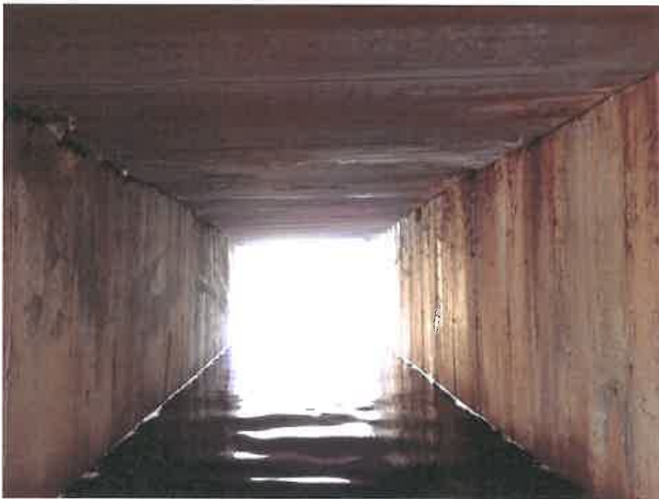
Photo No. 2 – Inside of Culvert
