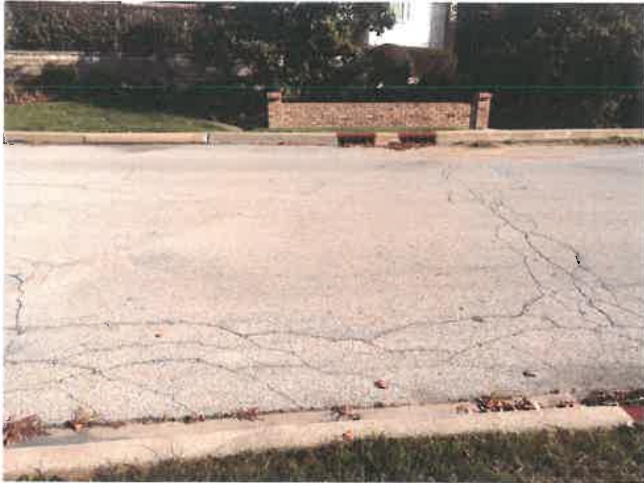
Photo No. 3 – Roadway (looking east)
