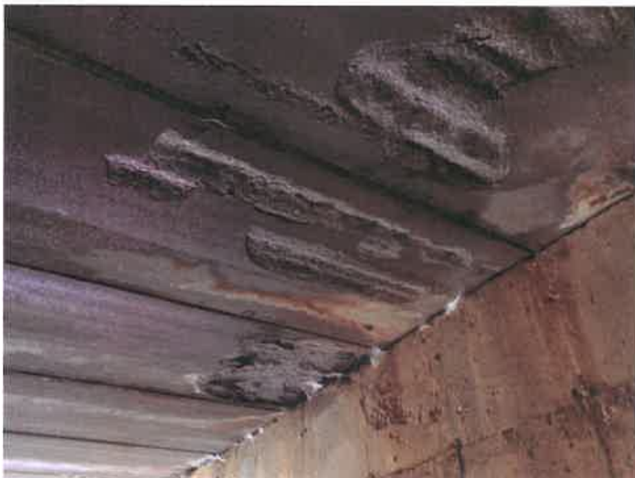
Photo No. 6 – Underside Precast Panels
