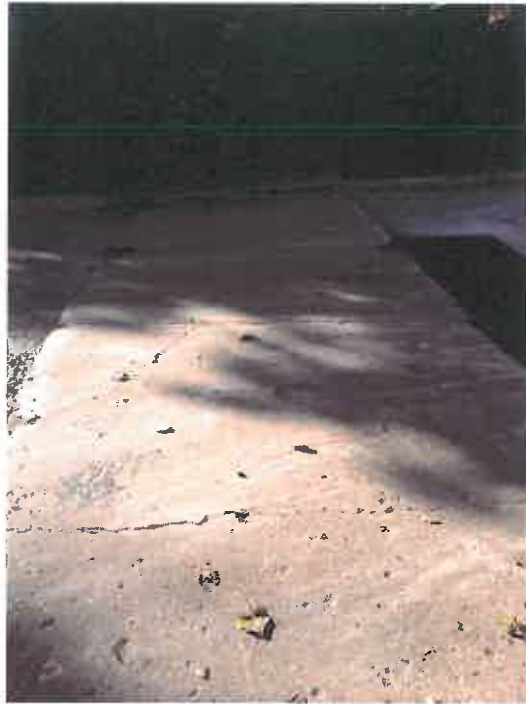
Photo No. 3 – Roadway Surface
