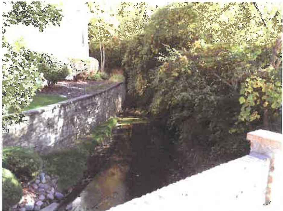
Photo No. 4 – Looking Downstream (looking east)
