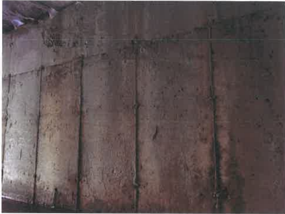
Photo No. 7 – Typical Wall Condition
