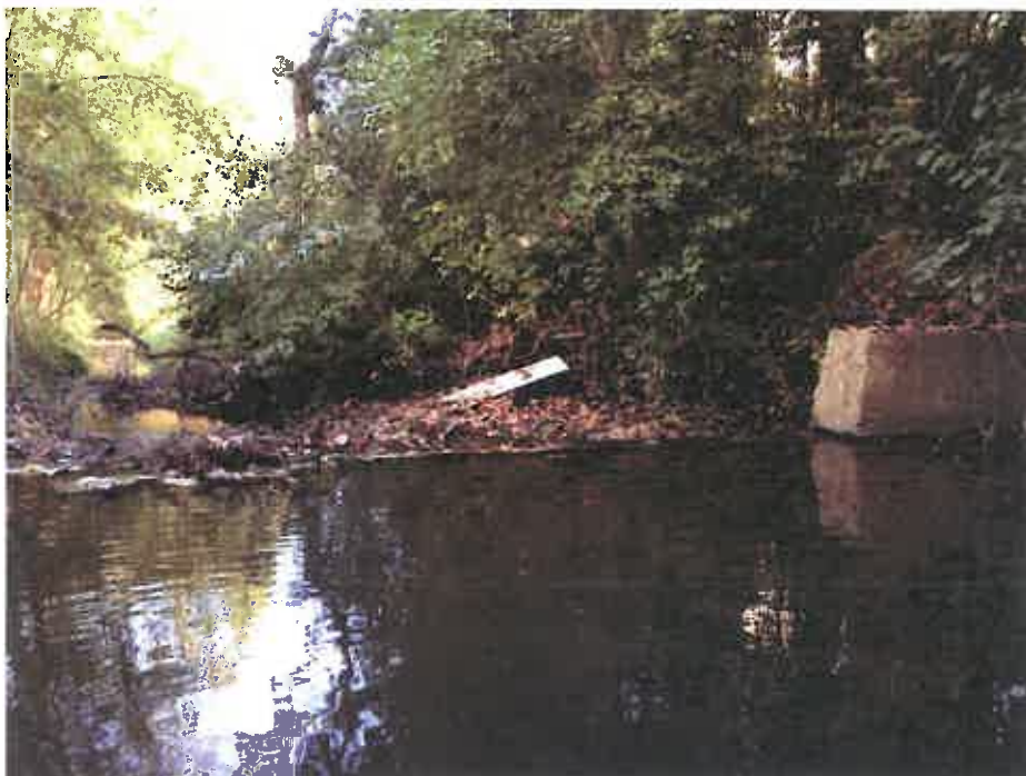
Photo No. 8 – Weir Downstream
