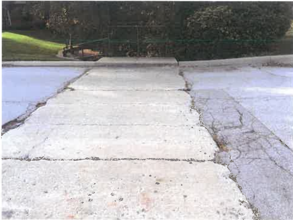
Photo No. 3 – Roadway Surface
