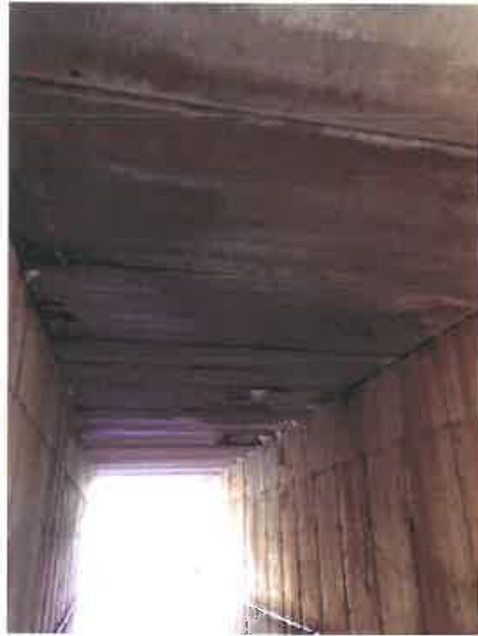
Photo No. 1 – Inside of Culvert
