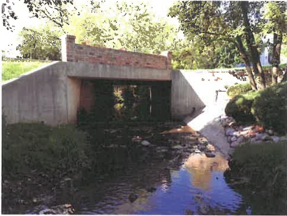
Photo No. 1 – East Elevation
