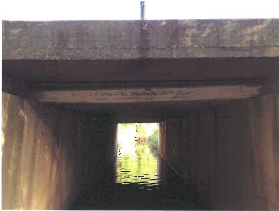
Photo No. 1 – Inside of Culvert
