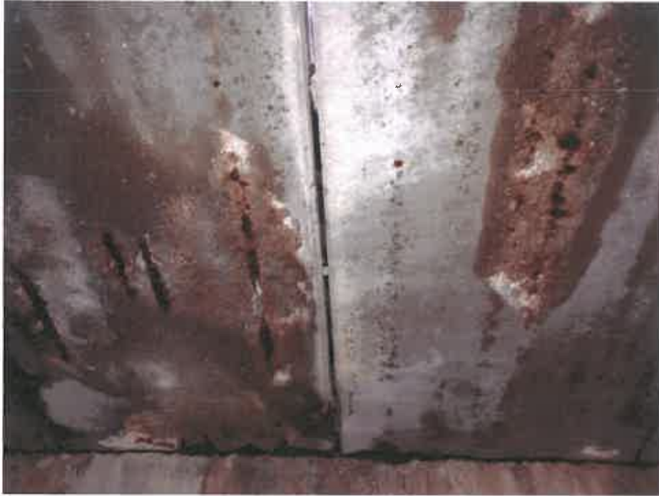
Photo No. 5 – Underside Precast Panels
