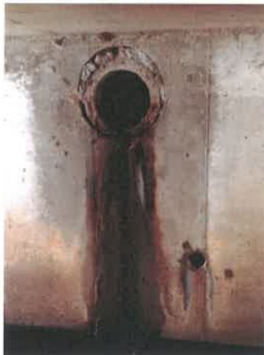
Photo No. 6 – Pipe Penetration
