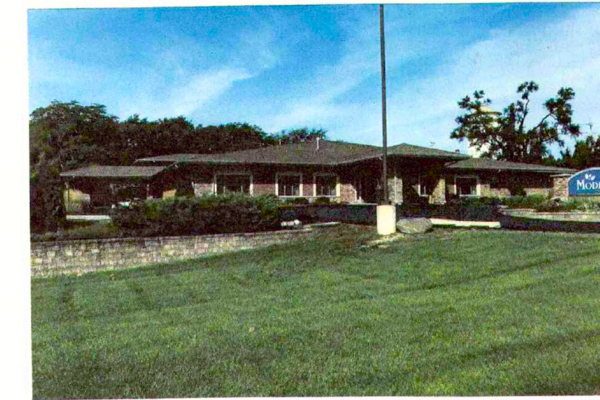
EAST WALL SOUTH END
