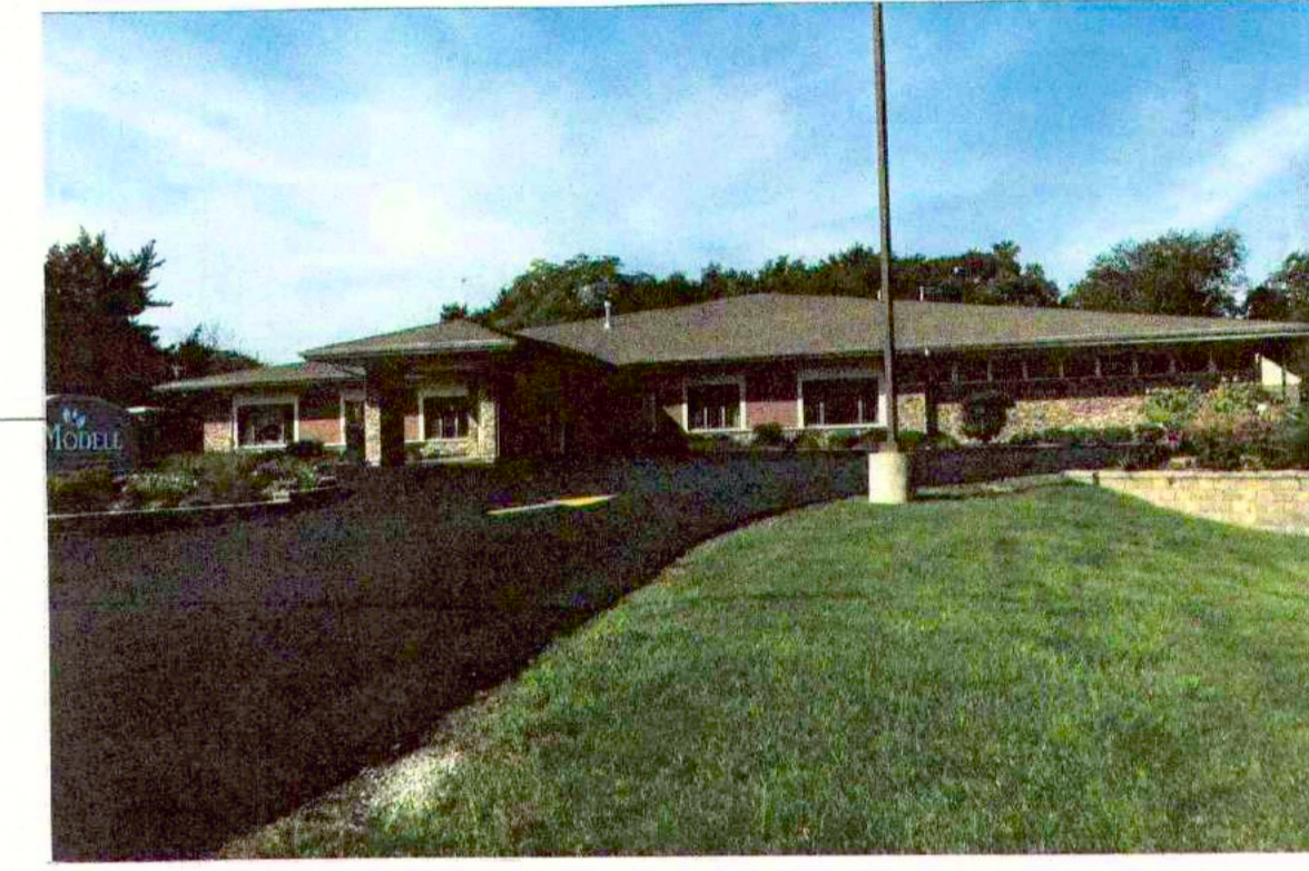
EAST WALL NORTH END
