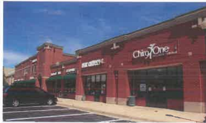
Figure C9.1a: Scale of signage is appropriate for building. Multiple signs are displayed in a consistent manner.
