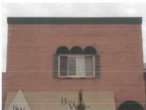
Fig. 28 Windows should be in scale with the other façade elements. Avoid windows which do not maintain rhythm of the wall as in this example
