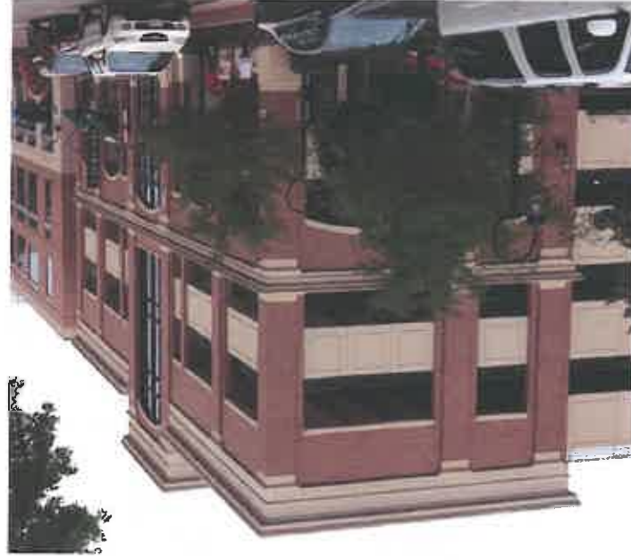
Figure C2.1a: Vertical brick articulation combines with horizontal stone/precast concrete banding to form overall grid frameworks. Cornices unify the top of the building.
