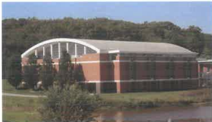
Figure C2.3: Effective use of modulation and horizontal articulation to minimize the appearance of bulk.
