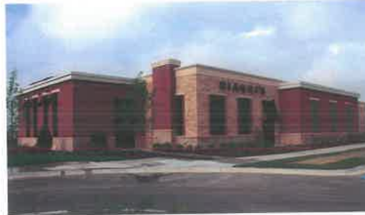
Figure C7.2: Secondary façade treated details and articulation that are consistent with the primary building faces.
