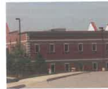
Figure C4.2a: AVOID extending vertical façade of a building face above the actual parapet or roofline to give the appearance of a false front. AVOID unscreened rooftop mechanical units.
