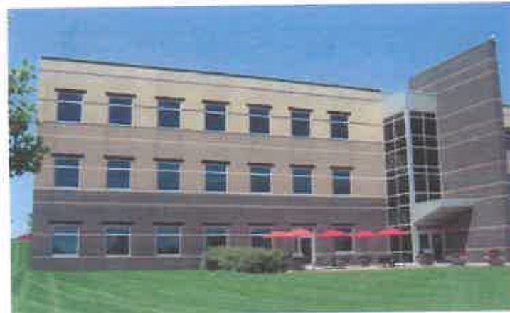
Figure B3.2: Entry is clearly marked by a tower feature, variation in color and material, canopy, and recess/projection.
