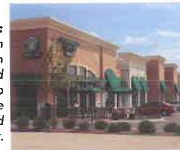
Figure C4.2b: Raised parapet with substantial depth creates varied rooflines. Rooftop mechanicals are completely screened by the parapet.
