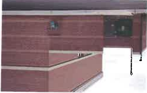
Figure C8.3: Refuse screening is discreet and consistent with the building
