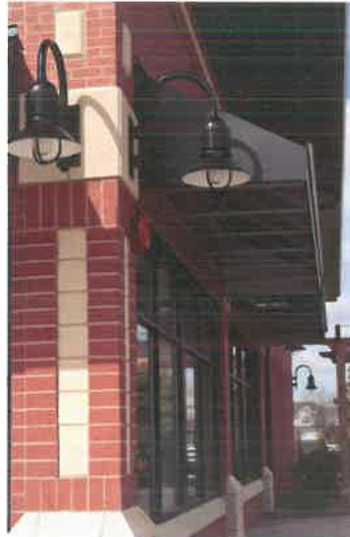
Figure B5.4: Patterned masonry detail and light fixtures enhance pedestrian character.
