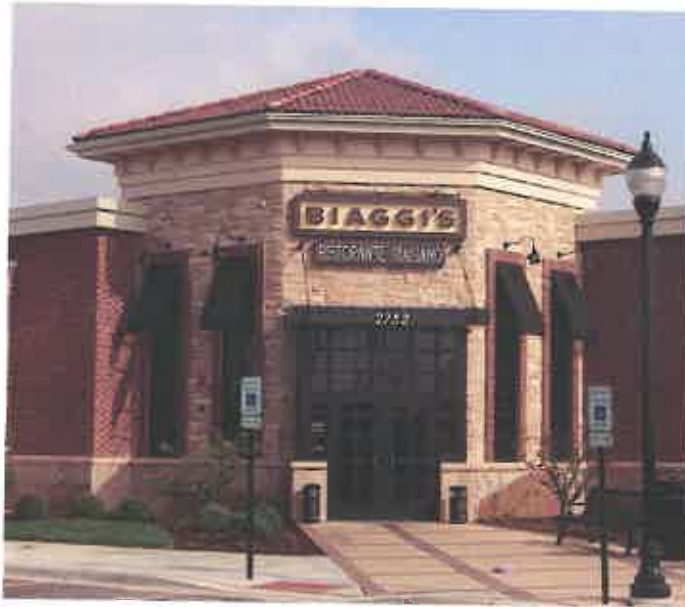
Figure B5.1 and 5.2: This building incorporates masonry knee wall and decorative cornice elements
