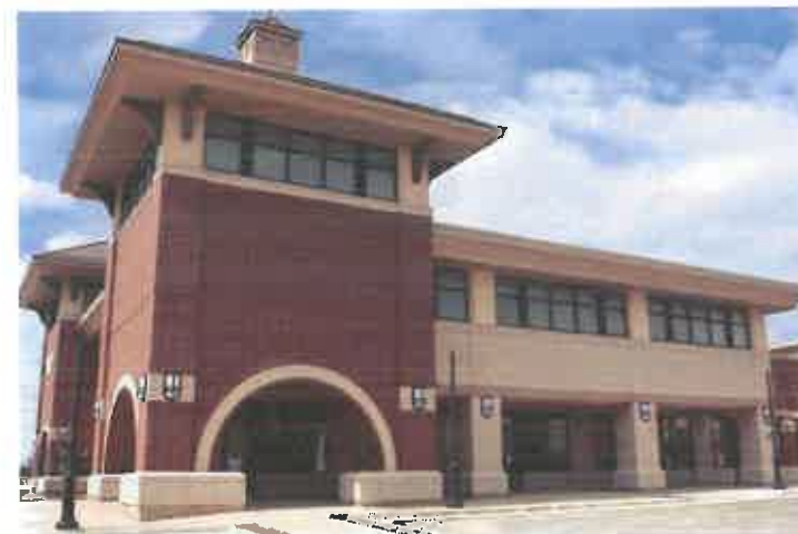
Figure C1.2b: Balance is created by tower on the left side offsetting the longer section to the right.
