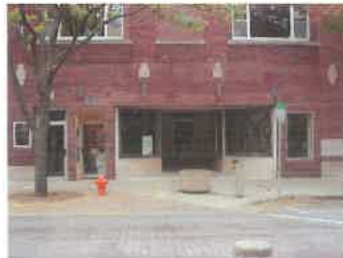
Fig. 14: Entries without detail and definition are unattractive and do not invite customers into the establishment. If entries are setback, extra care should be given to the detailing as in Figure 11.
