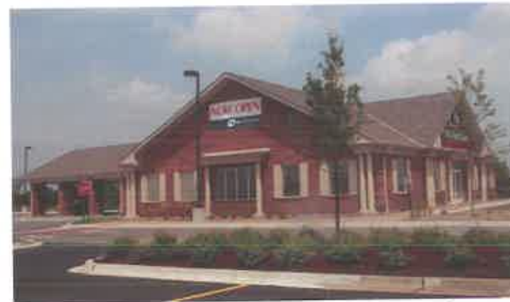
Figure C7.3: Secondary façade enhanced by use of varied rooflines, architectural detail that is consistent with front façade.
