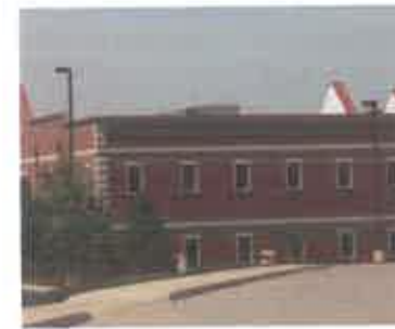
Figure C4.2a: AVOID extending vertical façade of a building face above the actual parapet or roofline to give the appearance of a false front. AVOID unscreened rooftop mechanical units.
