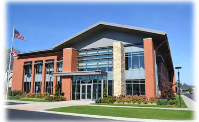
The above-pictured office building not only incorporates encouraged building materials, it has distinguished architectural details and a clearly defined entry.
