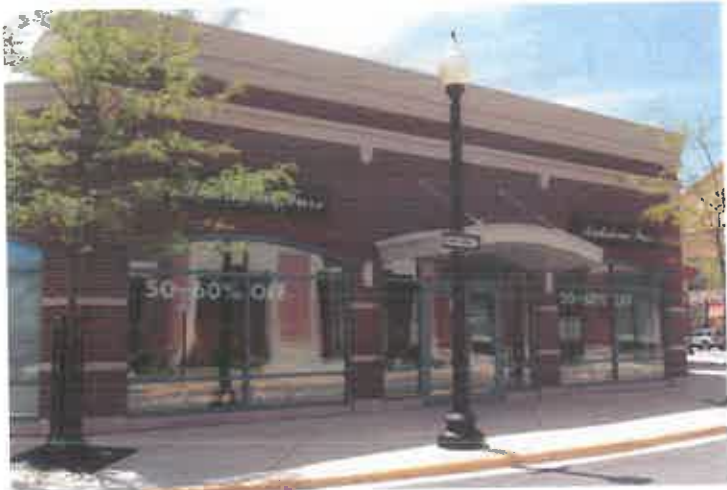
Figure B4.4b: Acceptable use of metal awnings
