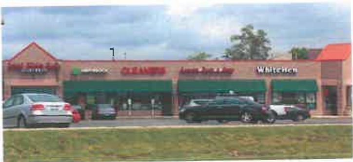
Figure B4.3 AVOID awnings extending over several windows and doors.
