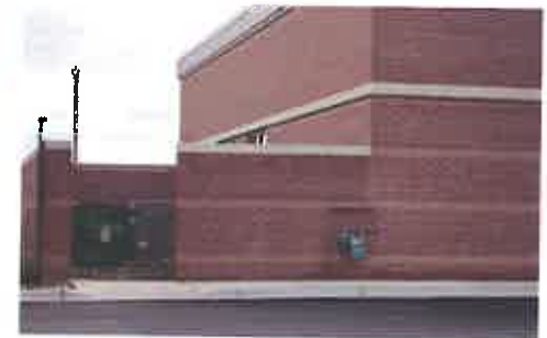
Figure C8.3: Refuse screening is discreet and consistent with the building
