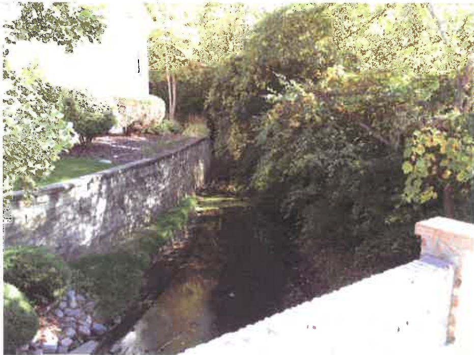
Photo No. 4 – Looking Downstream (looking east)
