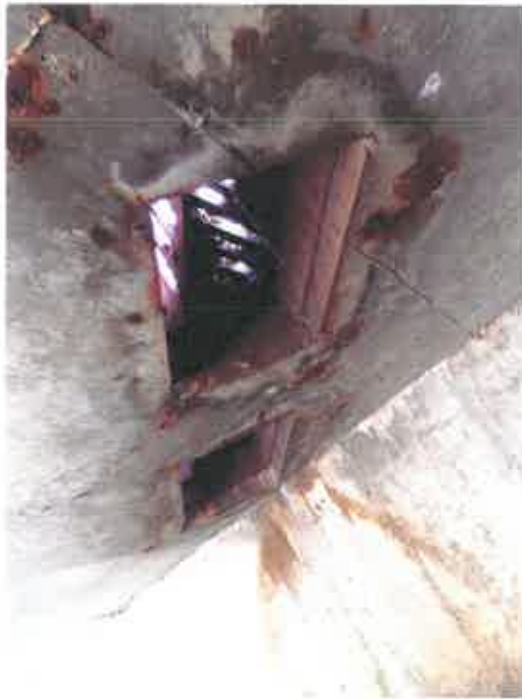
Photo No. 5 – Drains
