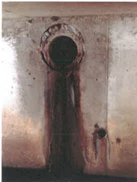
Photo No. 6 – Pipe Penetration
