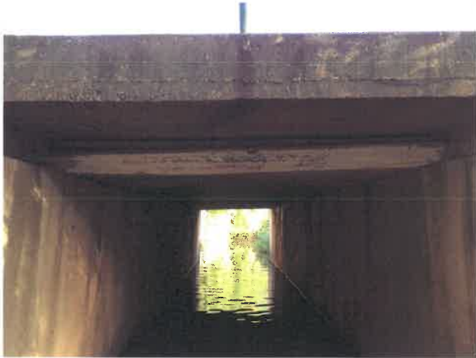
Photo No. 1 – Inside of Culvert
