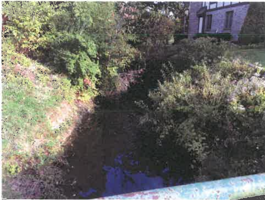
Photo No. 7 – Looking Downstream
