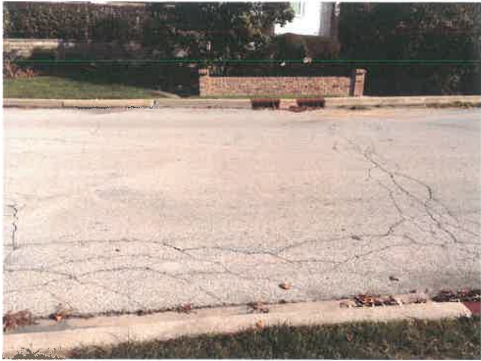
Photo No. 3 – Roadway (looking east)
