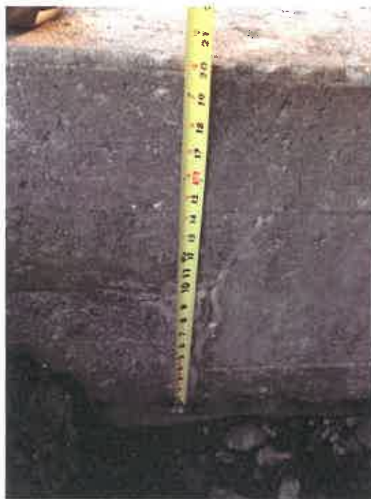
Photo No. 4 – Concrete Thicknesses
