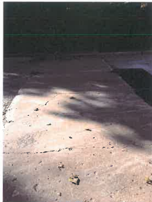
Photo No. 3 – Roadway Surface
