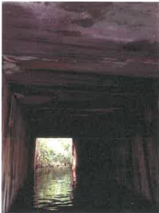
Photo No. 2 – Inside of Culvert
