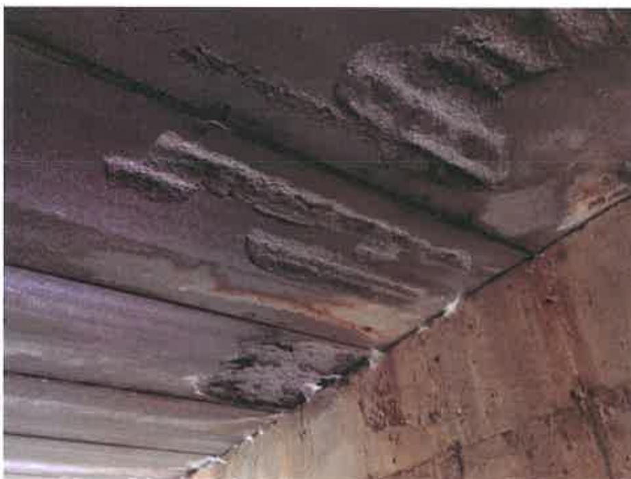
Photo No. 6 – Underside Precast Panels
