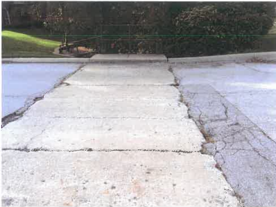
Photo No. 3 – Roadway Surface
