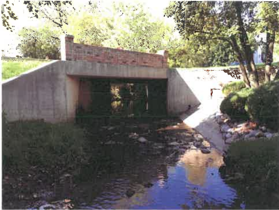
Photo No. 1 – East Elevation
