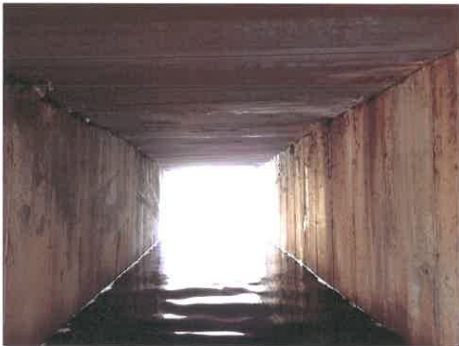
Photo No. 2 – Inside of Culvert
