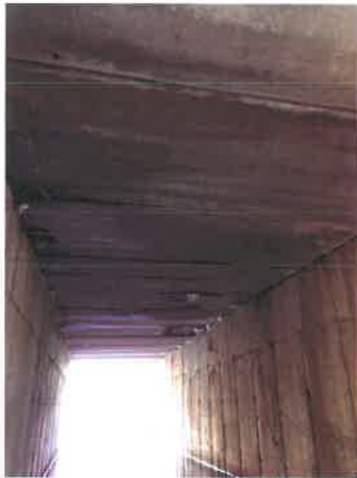
Photo No. 1 – Inside of Culvert
