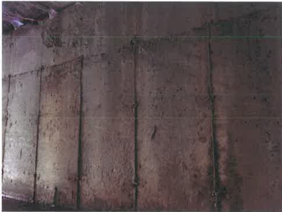
Photo No. 7 – Typical Wall Condition
