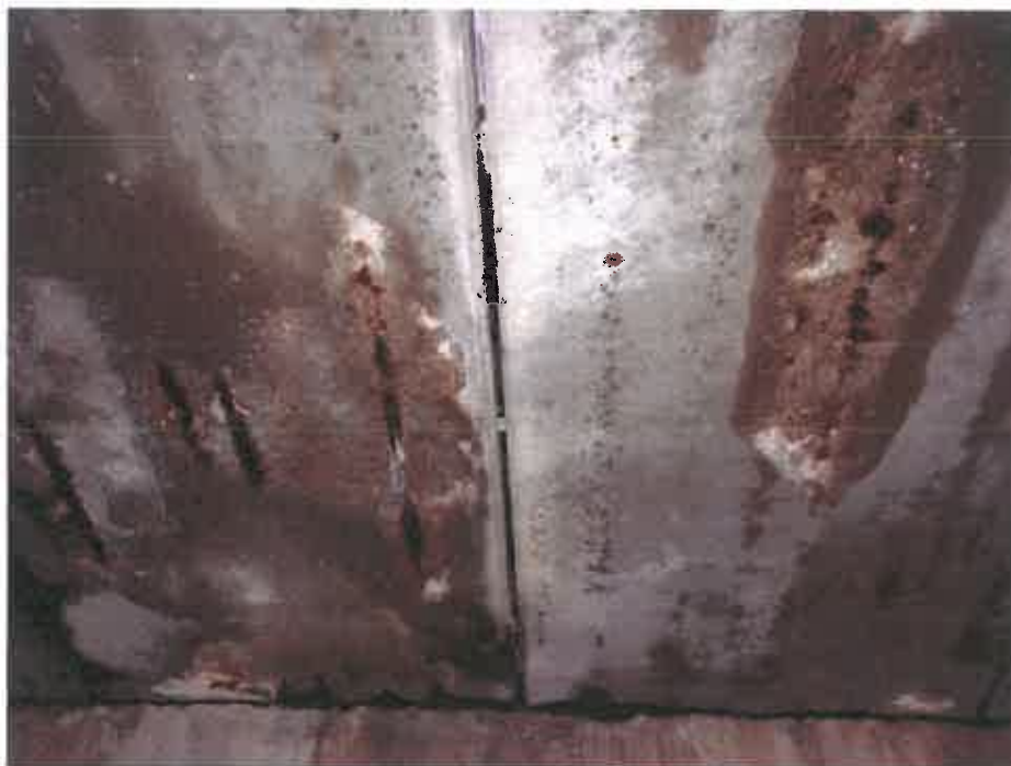
Photo No. 5 – Underside Precast Panels
