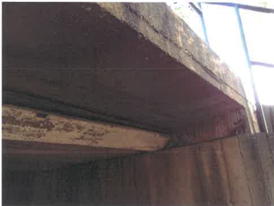
Photo No. 6 – Cast-in-place "sidewalk" on each end
