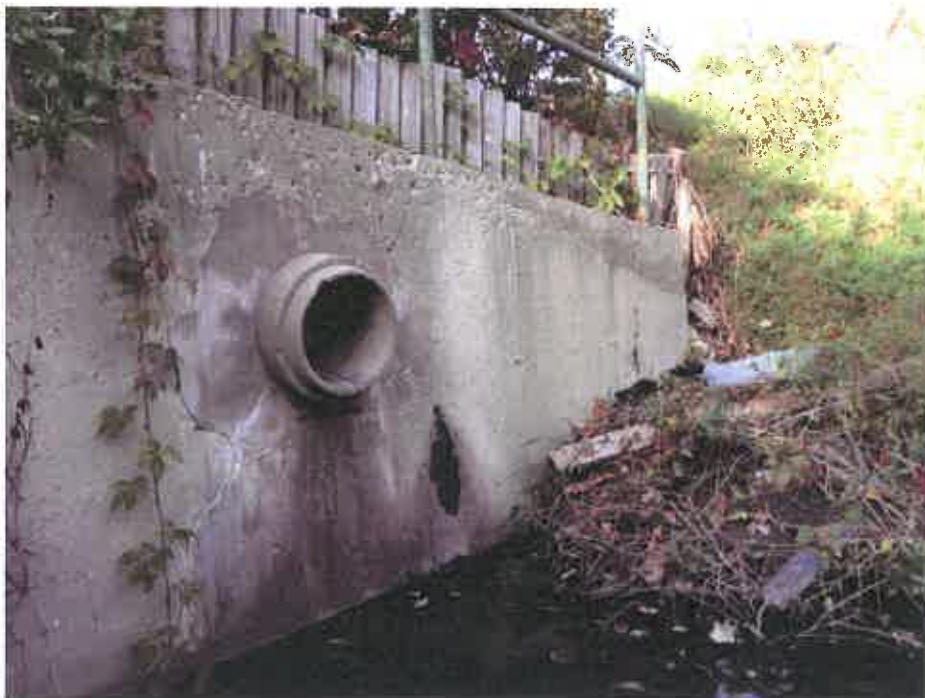
Photo No. 8 – Pipe Penetration
