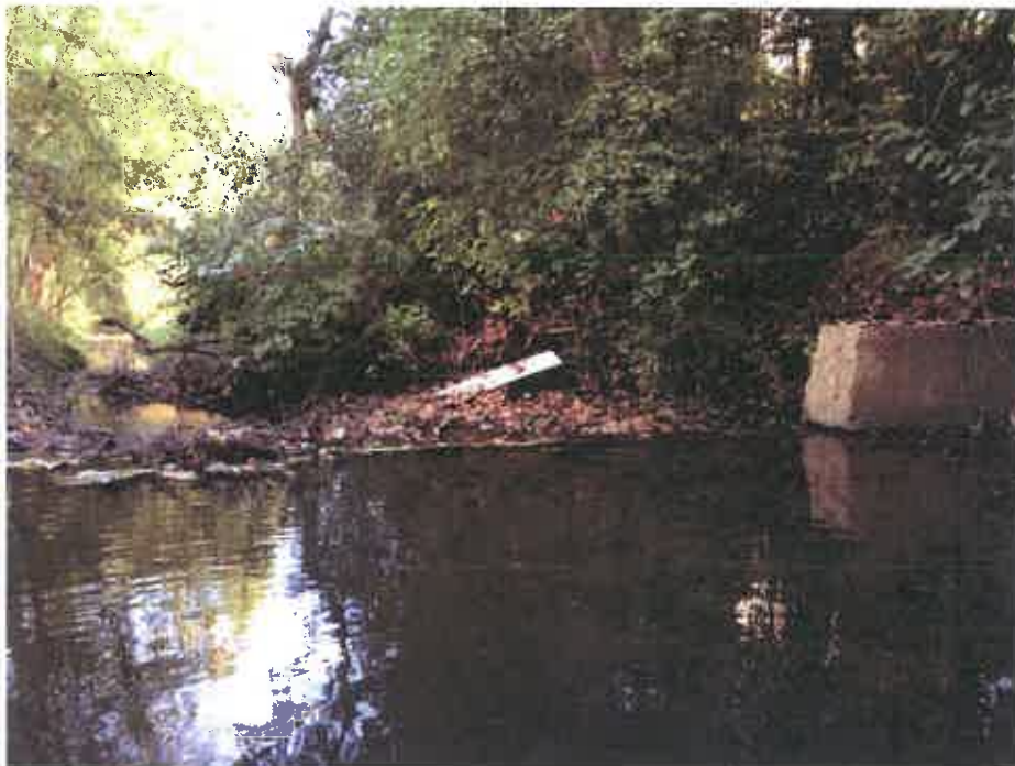
Photo No. 8 – Weir Downstream
