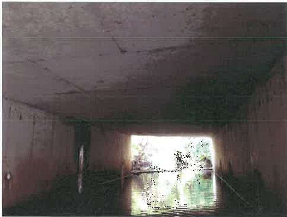
Photo No. 7 – Inside of Culvert
