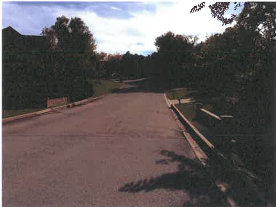
Photo No. 2 – Roadway Above (looking south)
