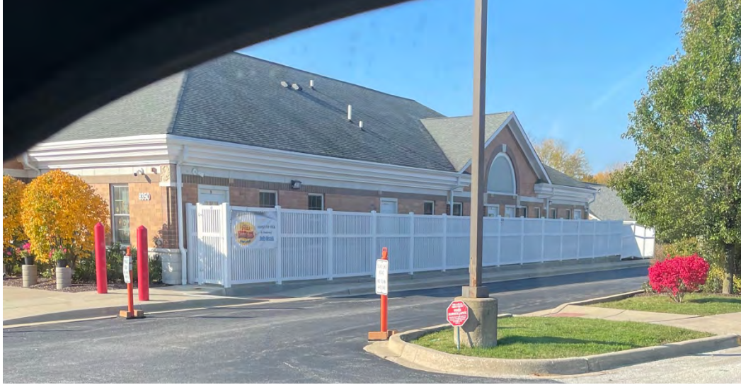
Goddard School (Daycare) 8350 Lemont Rd, Darien, IL 60561 – vinyl fencing / white, approximately 6 ft. high
