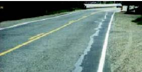
**Measure:** Accumulate the lengths along the surveyed lane of each type edge defect as it occurs. Divide the accumulated lengths by the length of the segment. Multiply by 100 to get percent, and round to a whole number.
