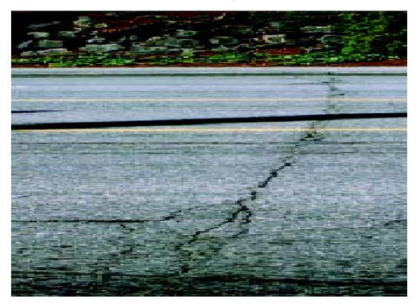
**Low** — The cracks have very little or no spalling along the edges and are less than 1/4-inch in width. If the cracks are sealed and the width of the crack prior to sealing is visible, they should be classified as Low Severity. (Good Prospect for Crack Sealing)
