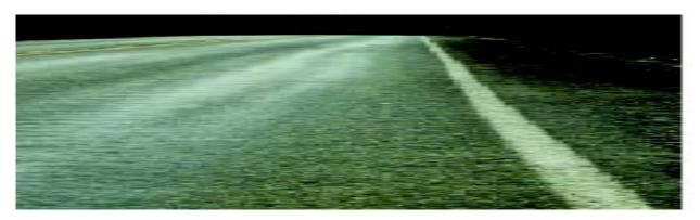
**Severity:** The severity of corrugation is defined as the maximum vertical deviation from a 10-foot straightedge placed on the pavement parallel to the center line of the roadway.
